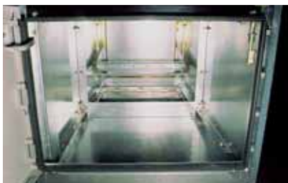
View of the feeder compartment with the metallic segregation sheet removed.
